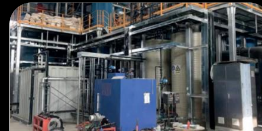
China BIONEX® Nitrate Removal Commissioning
