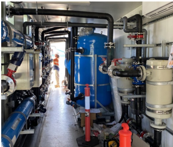
Koumala resin exchange drinking water plant under construction
